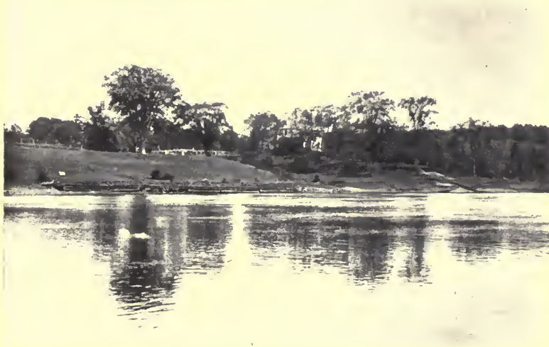
PIPE STAVE LANDING.
