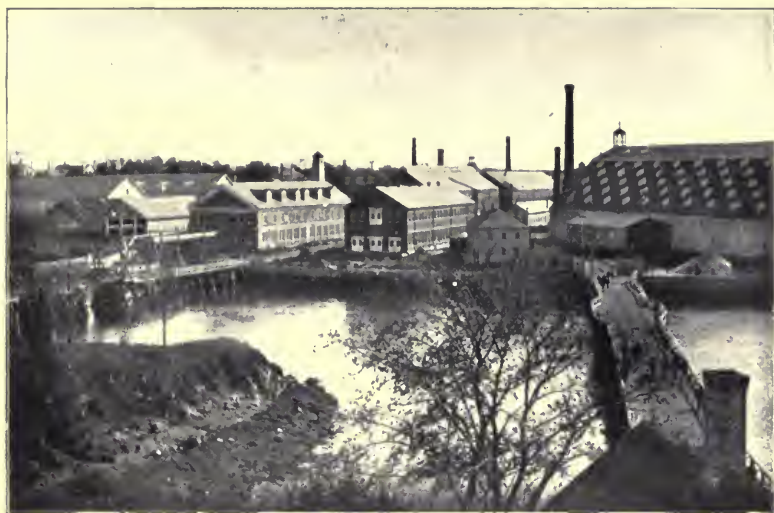
NAVY YARD BRIDGE.
