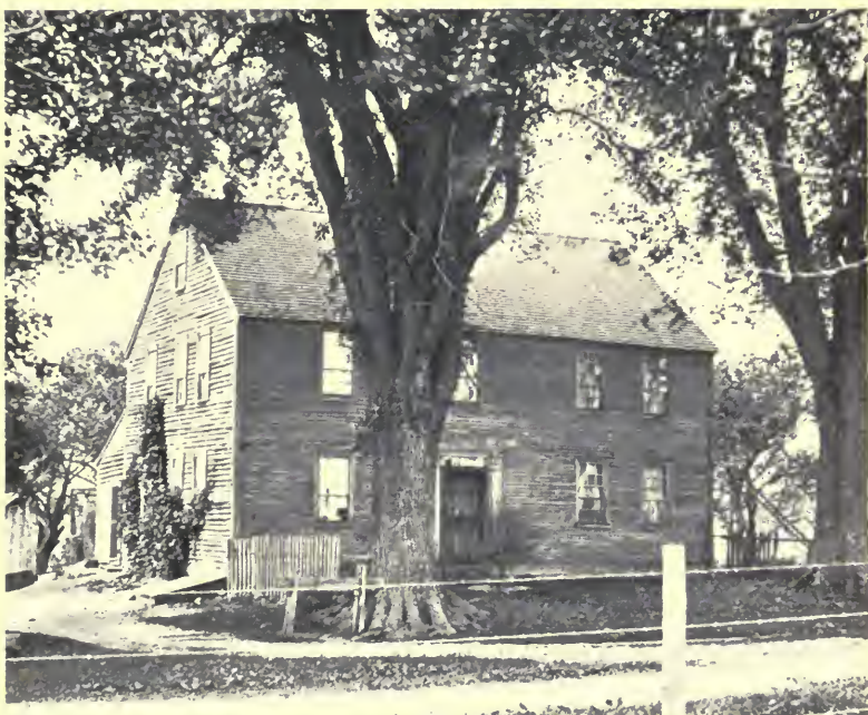
LEIGHTON HOUSE, BUILT BY JOHN LEIGHTON, 1690.
