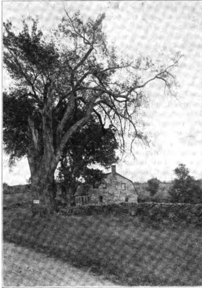
BRICK HOUSE BUILT IN WINDHAM, BY. COL. JEDEDIAH ELDERKIN, AN OFFICER IN THE CONTINENTAL ARMY, FOR HIS SON, AFTER THE REVOLUTIONARY WAR
