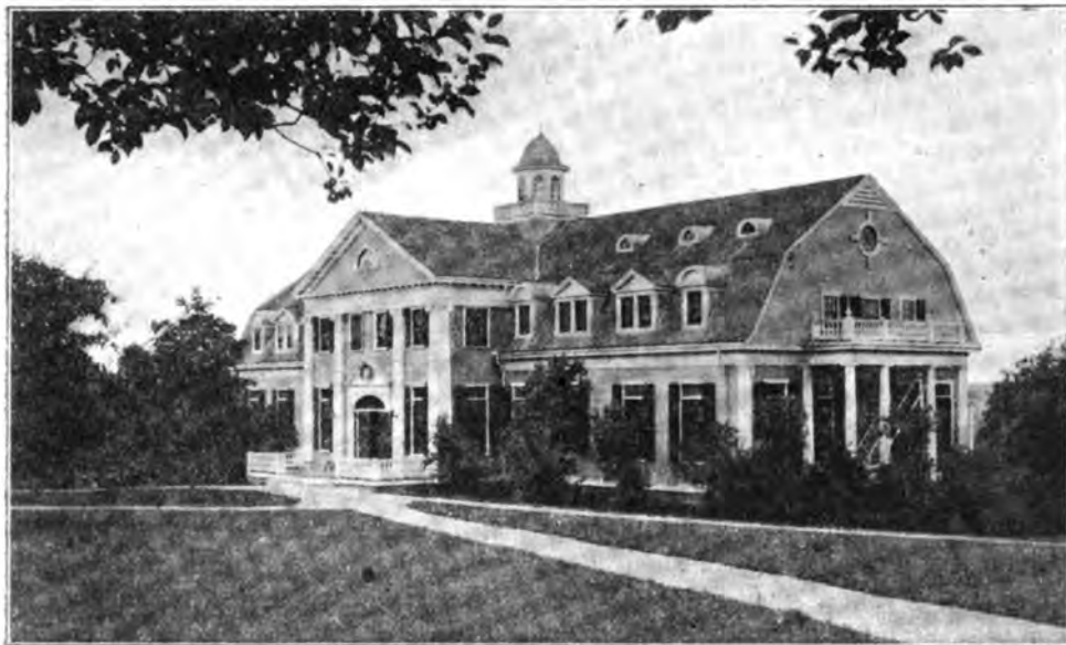
MAIN BUILDING, POMFRET SCHOOL
